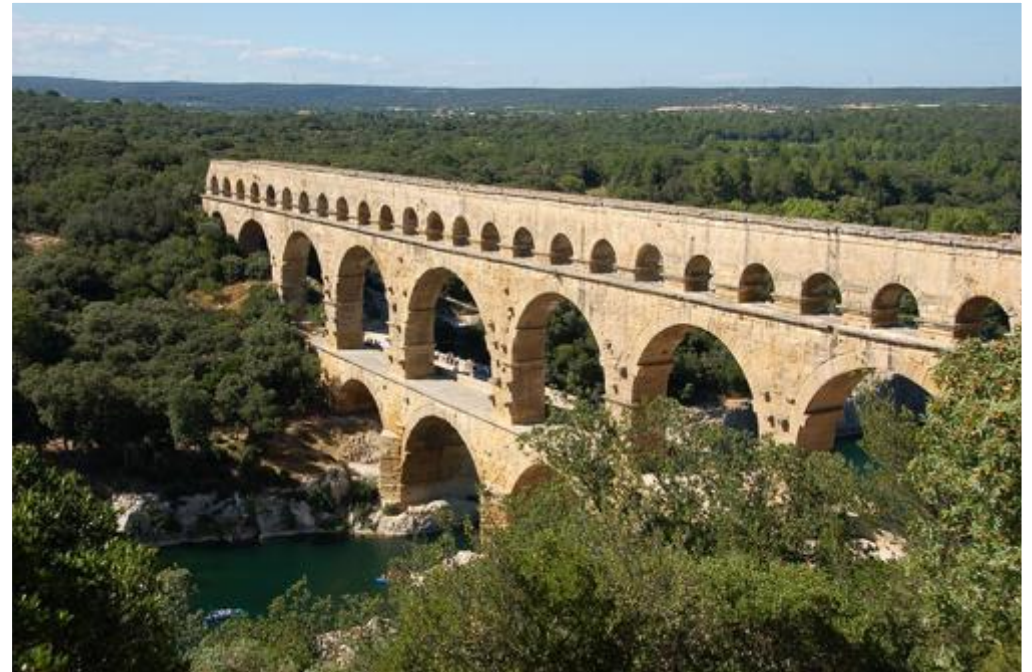
Pont du Gard in Southern France, one of the largest and best preserved Roman aqueducts. Photo: Wikicommons / Mimova.
